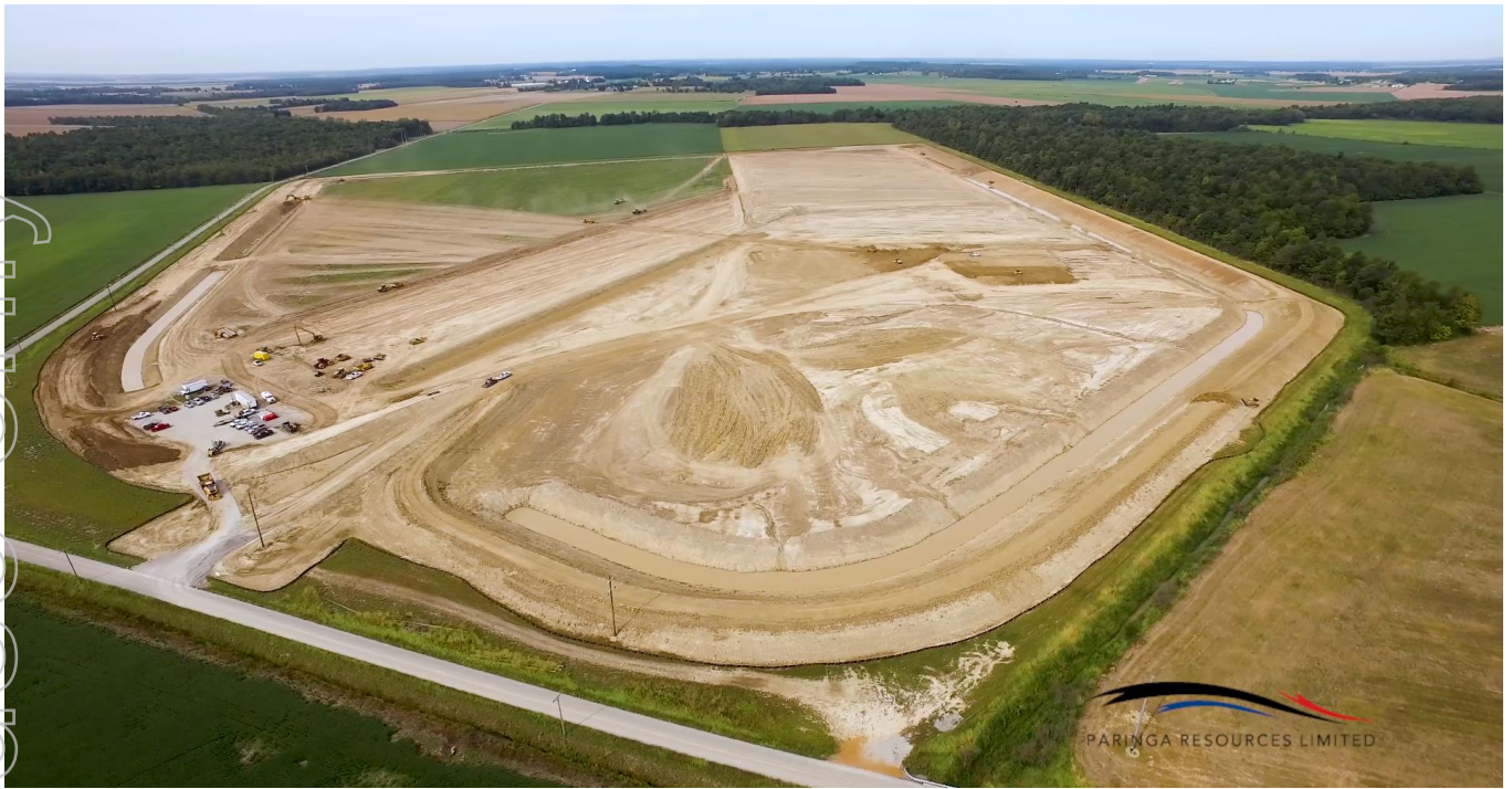
Mine Site Excavation and Development Continues at Poplar Grove Mine
