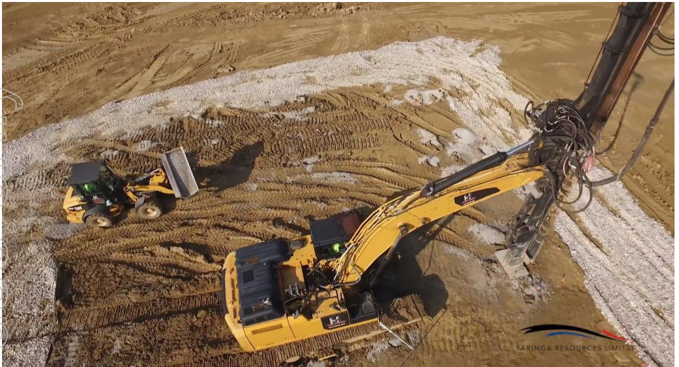
Preparing Foundations at the Preparation Plant at Poplar Grove Mine
