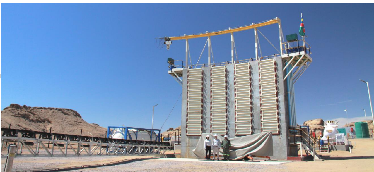
Figure 2: The Etango Demonstration Plant generated pregnant leach solution for IX testwork
