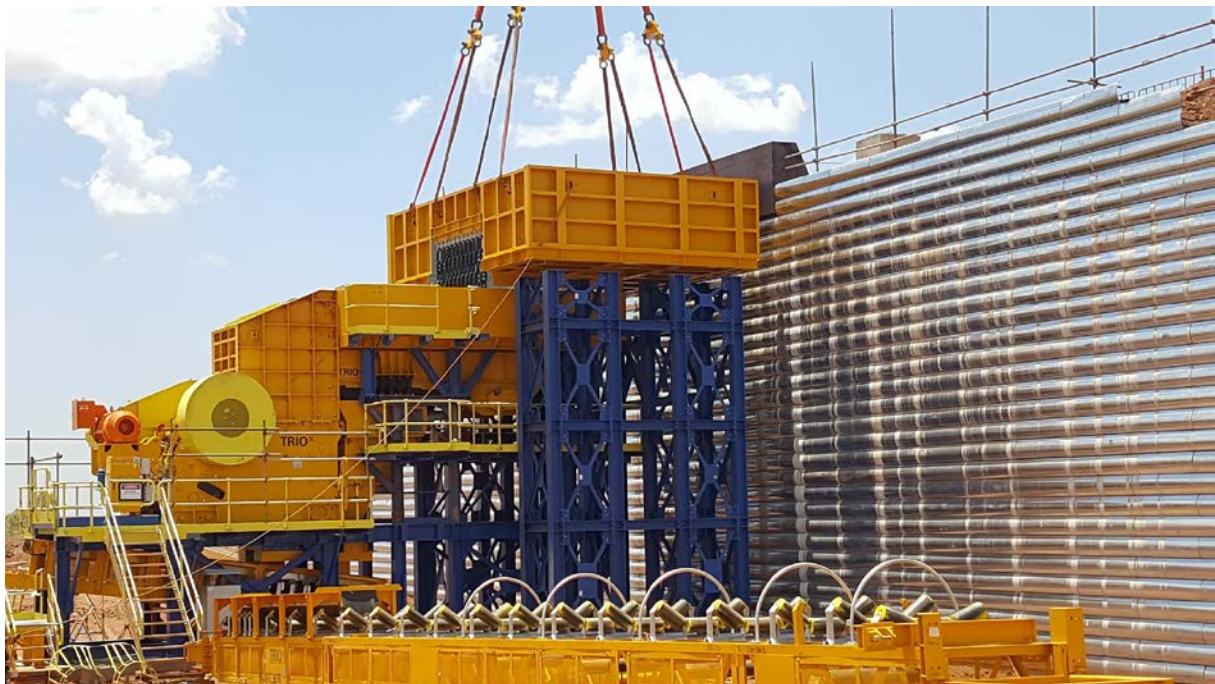
ROM Wall nearing completion
