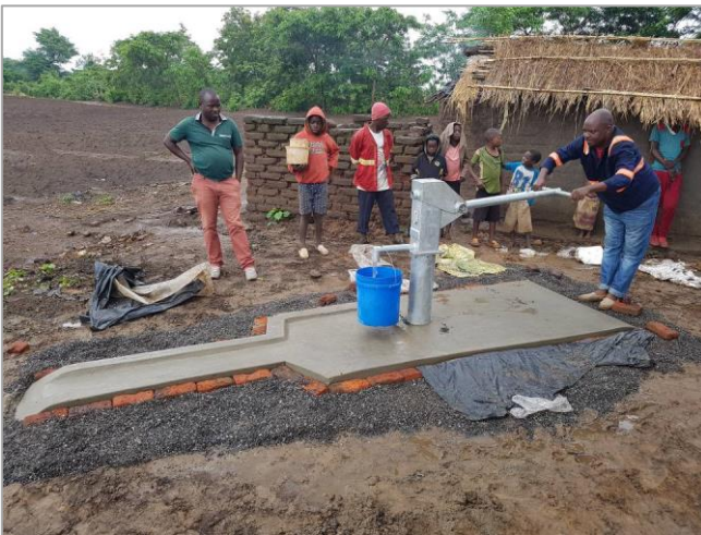
Figure 2a (LHS): Newly constructed water well with hand pump installed being tested for water yields.
