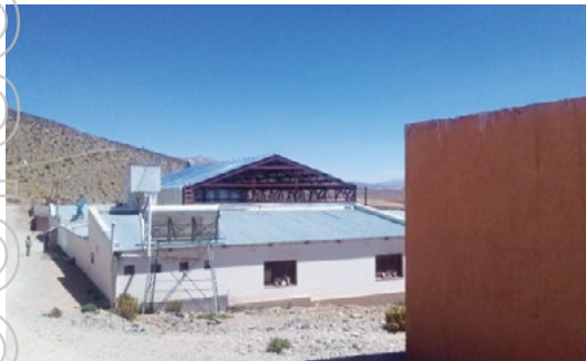
New roof, Olaroz Primary School
