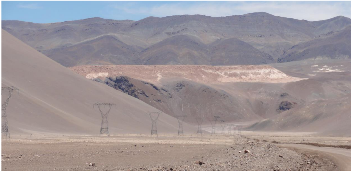
Figure 5: Existing electricity infrastructure along the road to Maricunga
