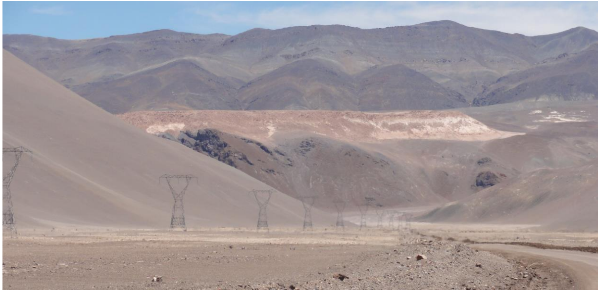
Figure 6: Existing electricity infrastructure along the road to Maricunga
