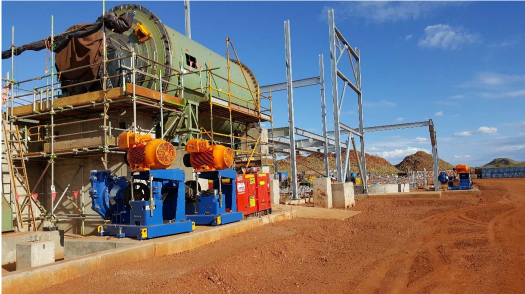
Ball Mill trunnion ends now installed
