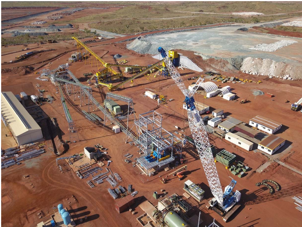
Mine site works near completion on the Altura Lithium Project
