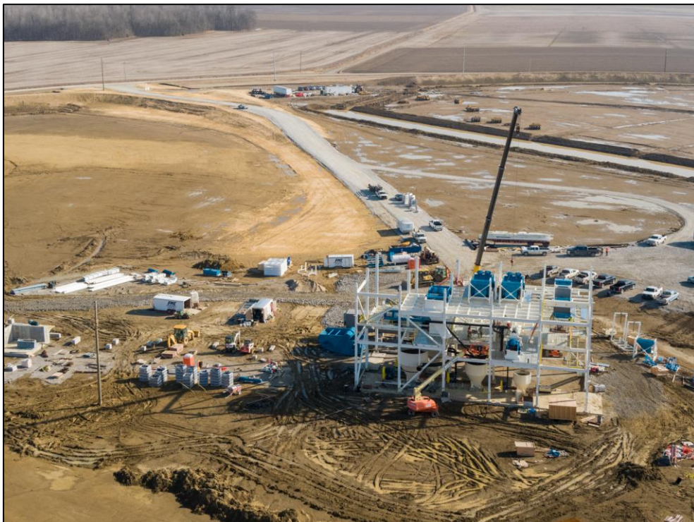
Installation of Infrastructure at the Preparation Plant
