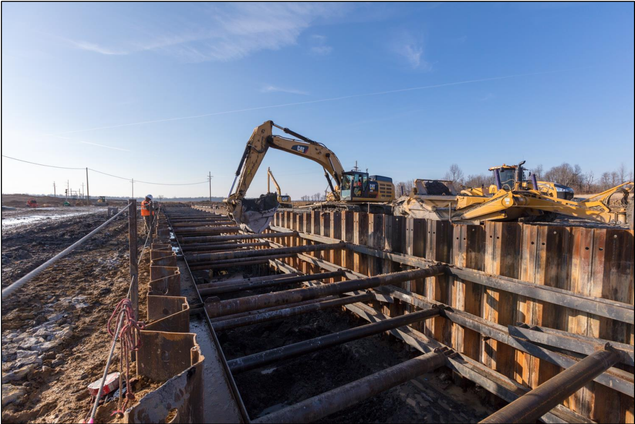
Construction of the Slope Portal to Access Underground Coal
