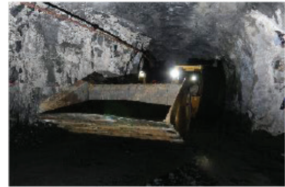
Existing underground haulage
