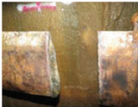
Location of removed section from underground bunton
