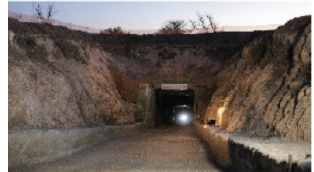
Surface portal access
