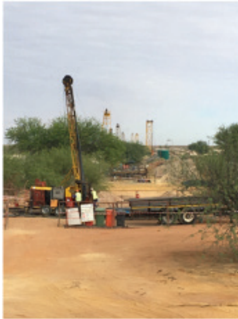
Drill rigs remain active on surface
