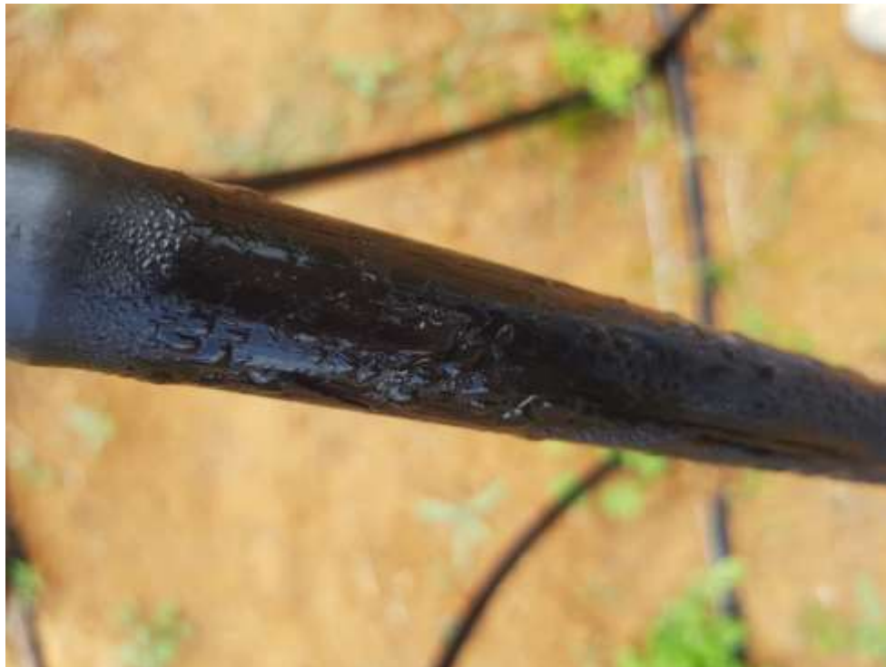
Condensation forms on the external surface of the pipes that flow by gravitation to the soil and roots.
