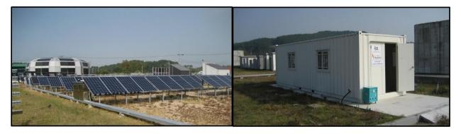
Figure 1: 20kW solar PV integrated with two 25kW V-KOR battery and the electricity grid in a field test site at Seosan-si in Korea.
