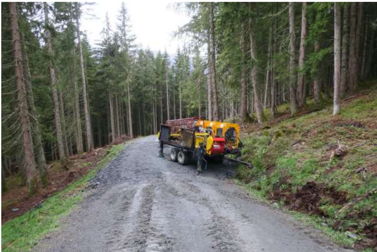
Figure 3 – Rig 2 setting up morning of 3 rd October, drilling end of day
