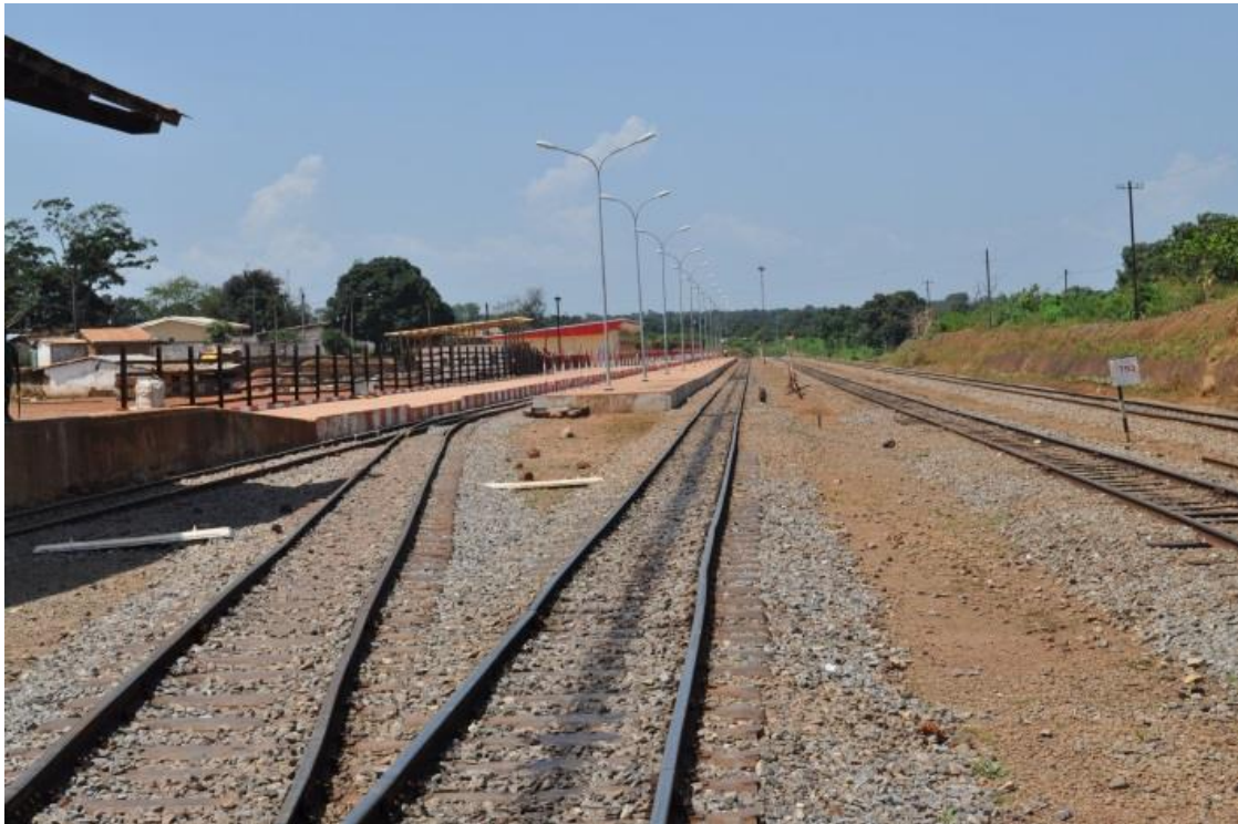
Figure 7: Rail station at the town Ngaoundal, near the Minim Martap Project
