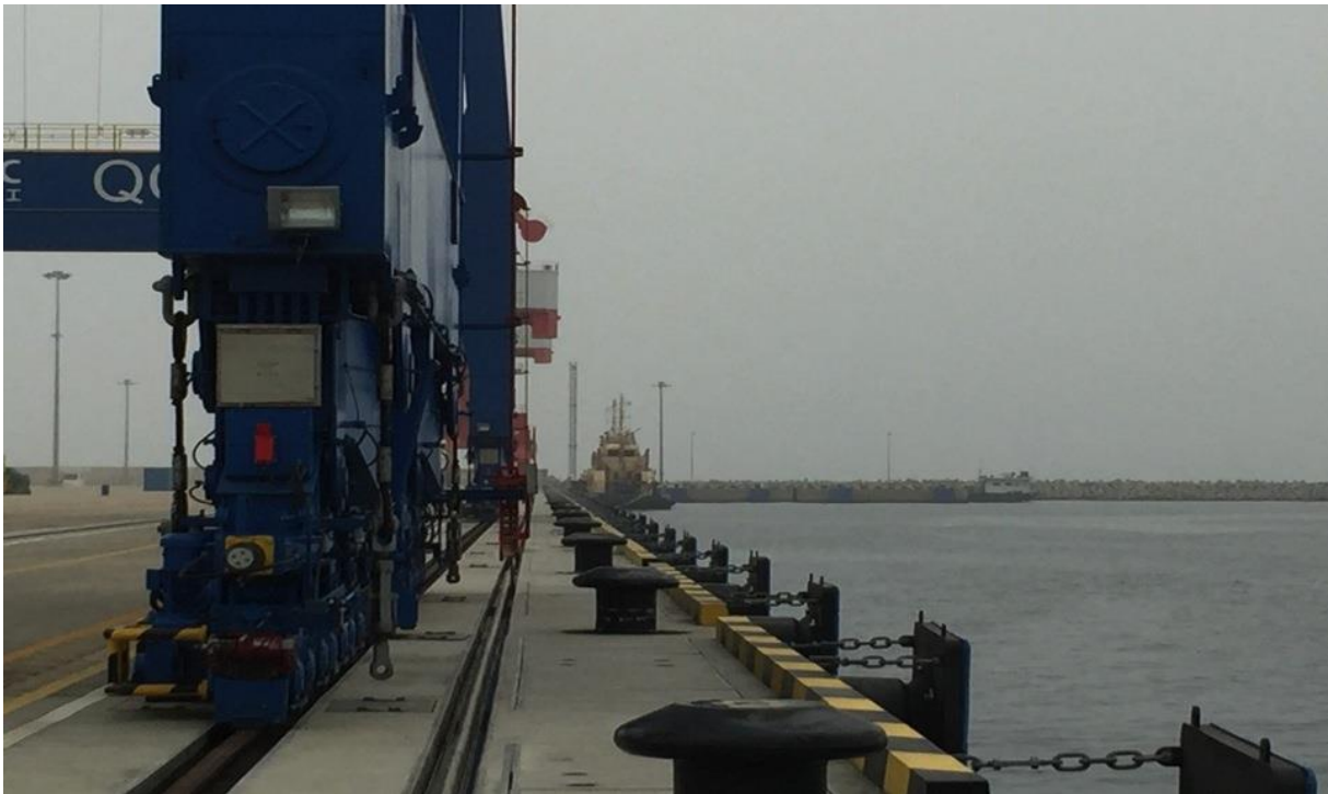
Figure 9: The wharf and ship berthing area of the Kribi Deep Sea Port
