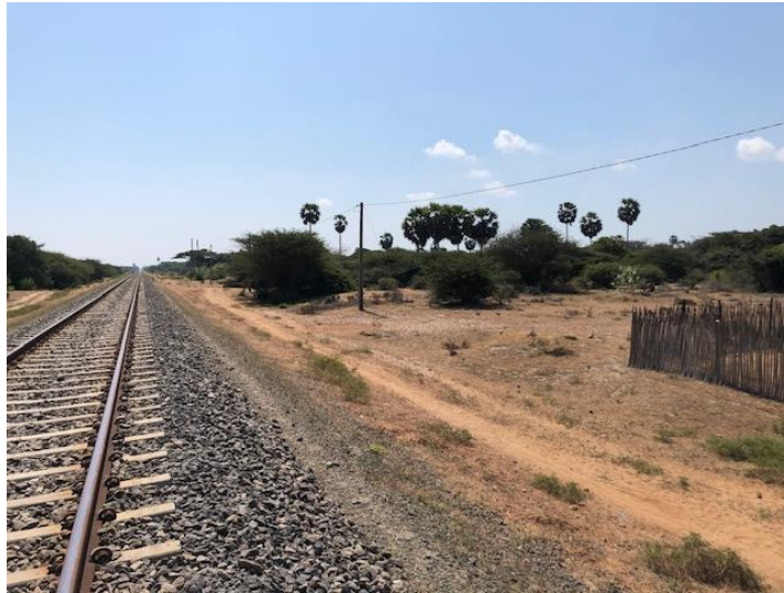
Newly refurbished rail track through the centre of Mannar island that links with the mainland rail system.
