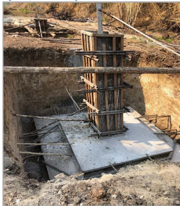
Figure 7 | Tower Footings on Okvau PDA
