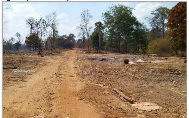
Figure 4 | Site Clean Up
