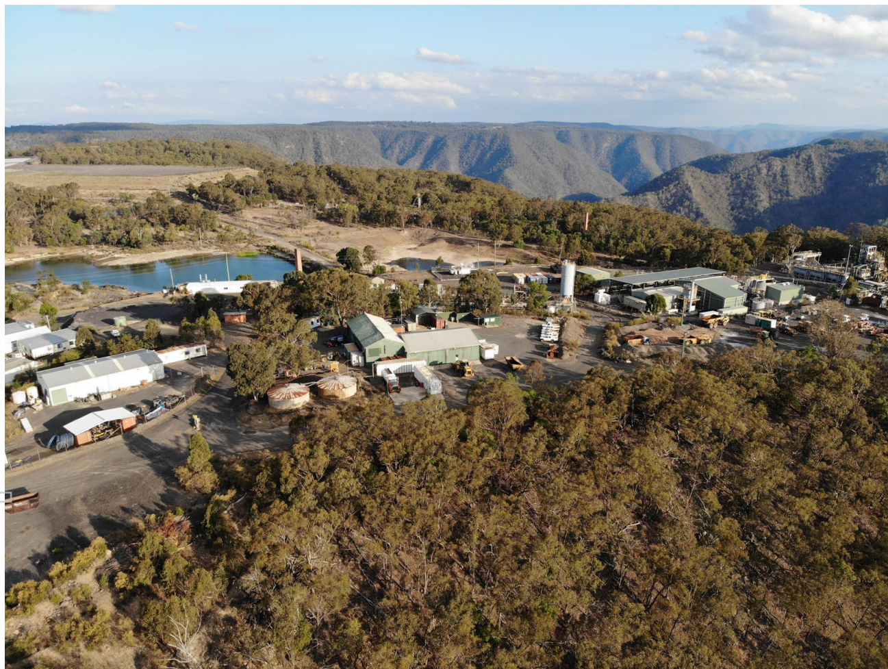
Figure 1 Hillgrove Gold-Antimony Project Site, showing processing infrastructure and layout
