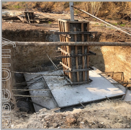
❑ Tower Footings on Okvau PDA.
