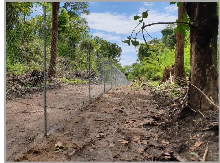
❑ Okvau PDA Fencing Complete.
