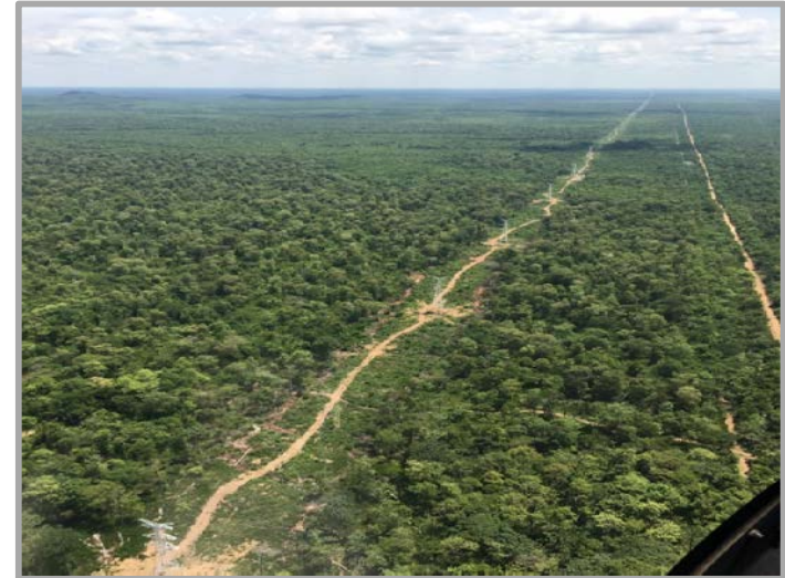
❑ Aerial View Powerline Towers & Corridor nearing completion, and will be available well ahead of site requirements.
