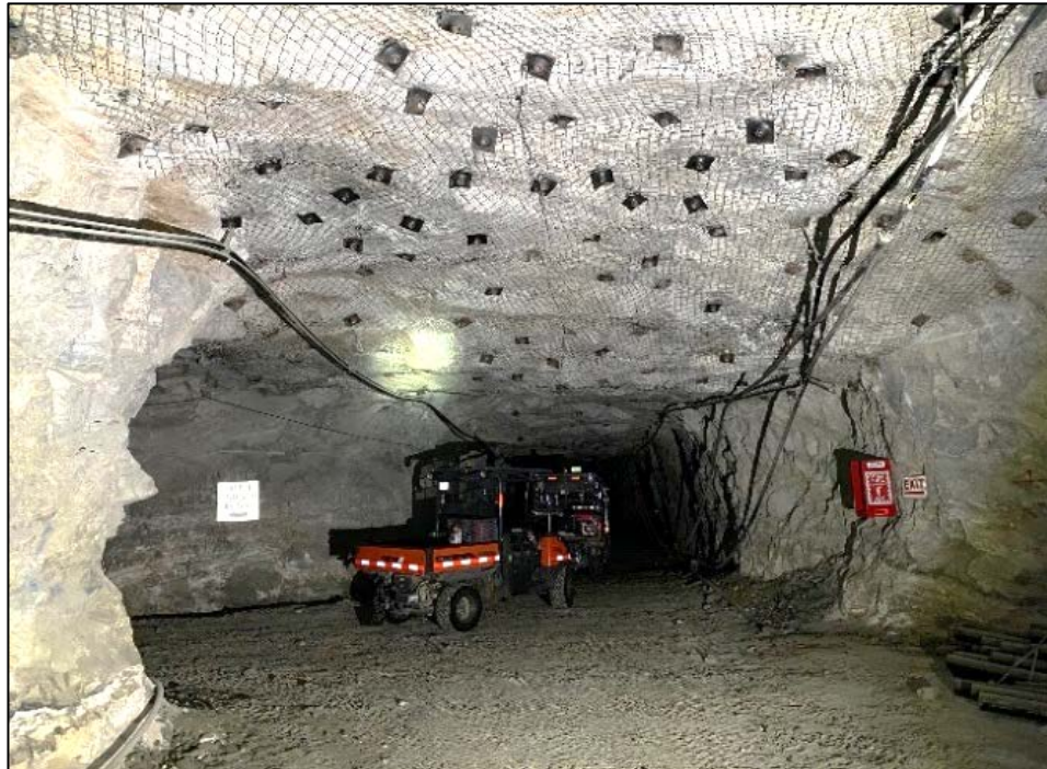
Underground development, showing the ground in good condition
