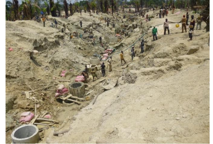
Artisanal mining through steel reinforced concrete wells on AG deposit on 17/3/2014
