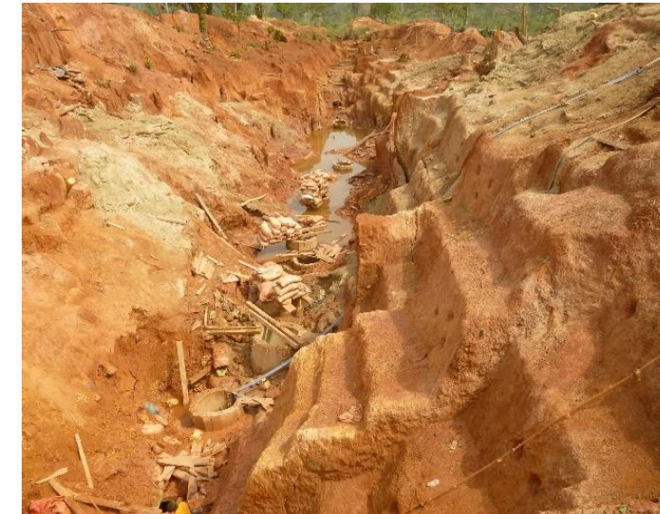
Steel reinforced concrete wells used at Gamina South on 15/12/2014 (Northern end of Abujar Middle tenement)
