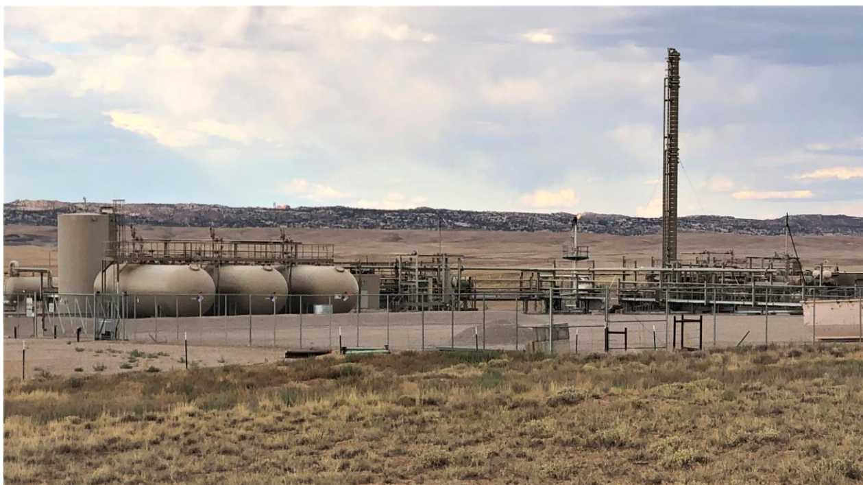
Figure 4: Existing natural gas conversion plant at Blue Hills
