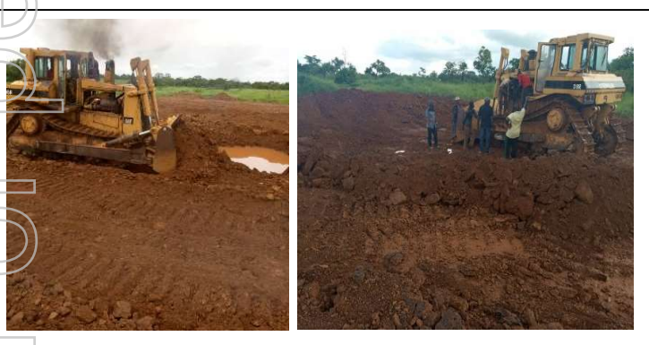
Laterite, iron ore and overburden removal (LHS).
