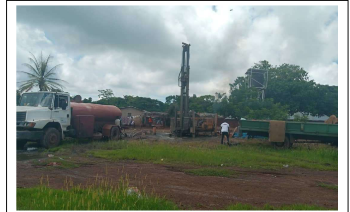
Drilling rig and support vehicles arrive on Irimi – Okpaka site.
