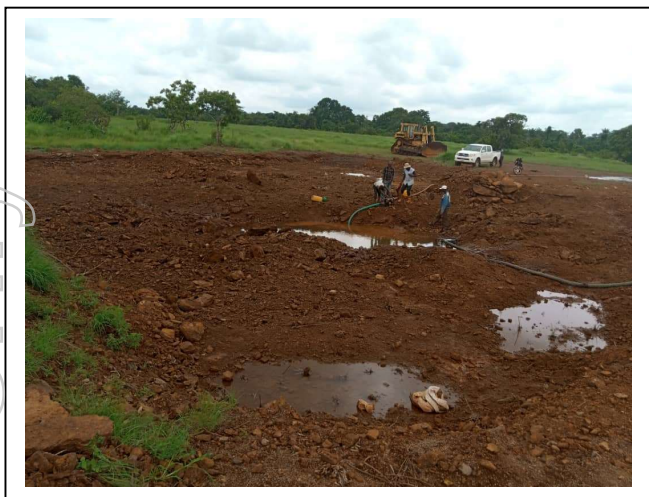
Dewatering sumps in preparation for re-start of trial mining
