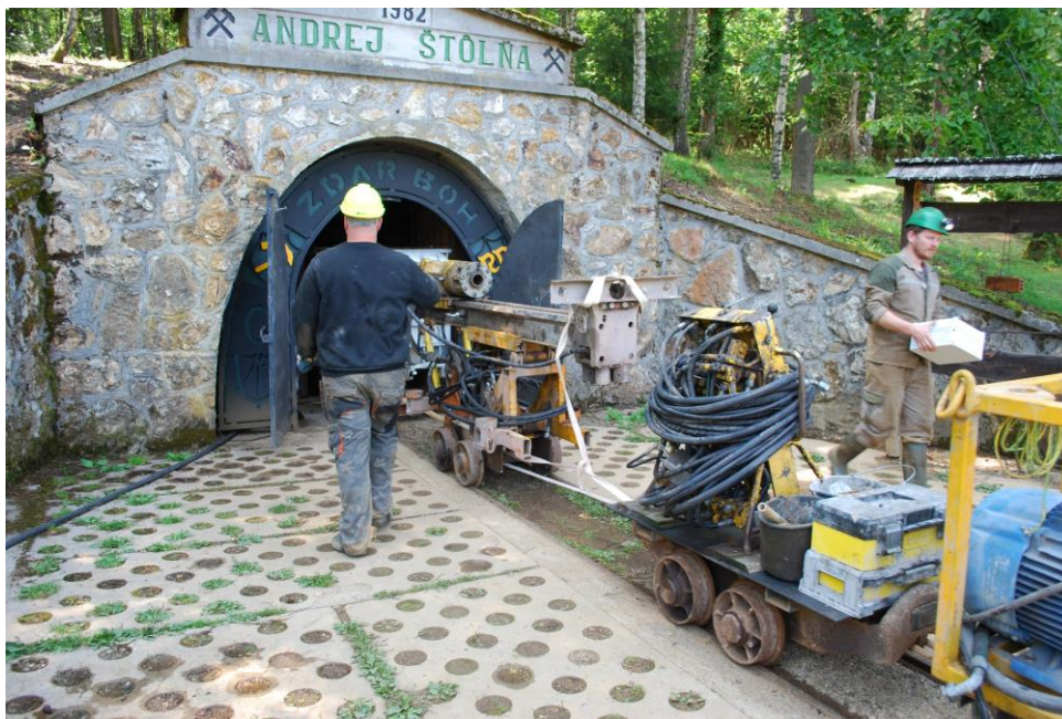
Image 1: Drill rig and ancillary equipment at the entry to the underground Andrej adit
