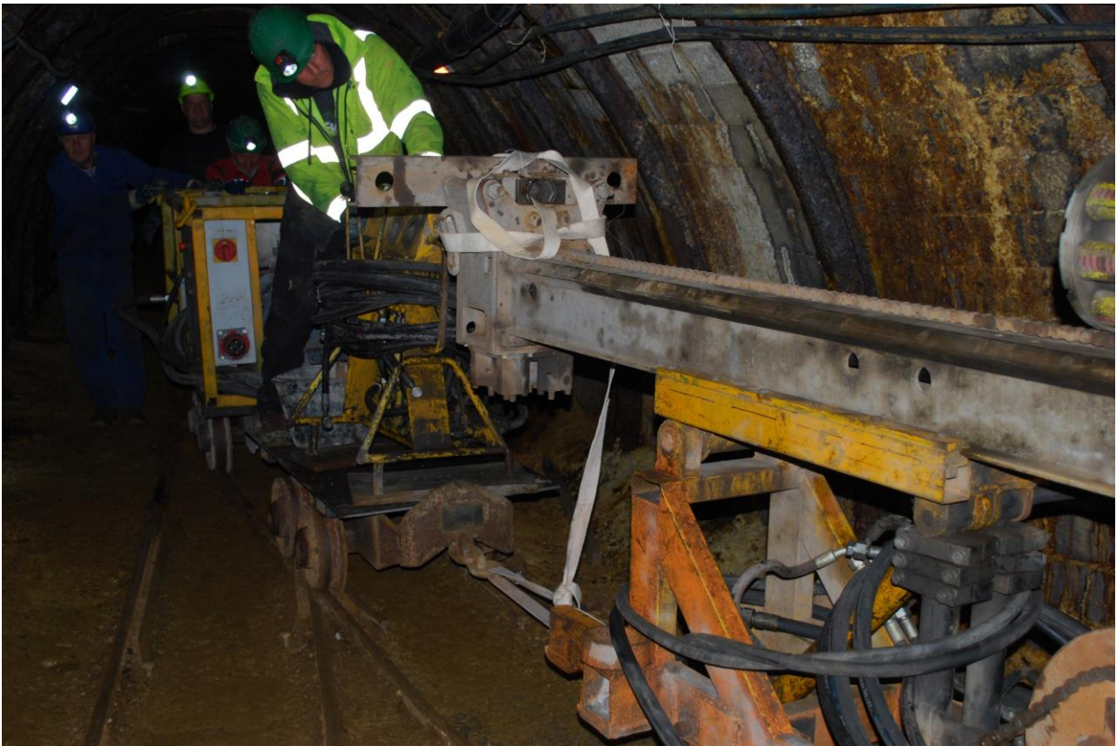
Image 3: Drill rig and ancillary equipment being mobilised to the underground Andrej adit
