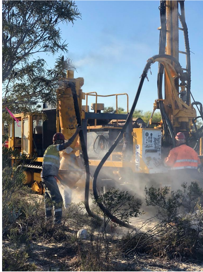
Commencement of 32 Hole Air-Core Drilling at Beharra
