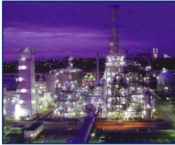
Negishi, Japan Built in 2003 342 MW
