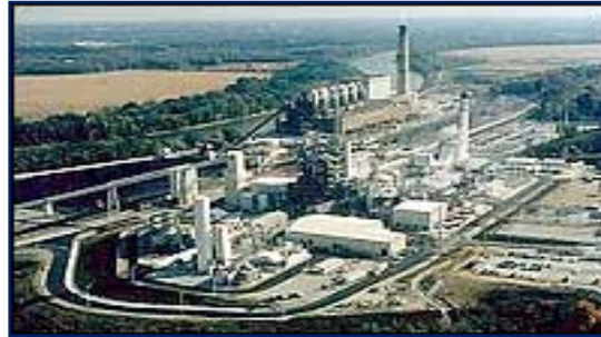
Wabash River Power Plant Indiana, USA Built in 1995. 262 MW
