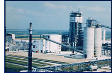
Tampa Electric's Polk Power Station Florida, USA Built in 1996. 250 MW
