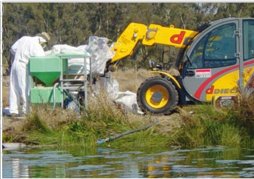
Preparing to apply Phoslock at a Waste Water Treatment Plant
