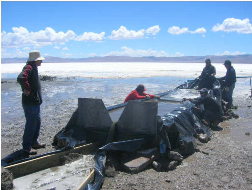
Preparing a V-notch weir for flow rate testing
