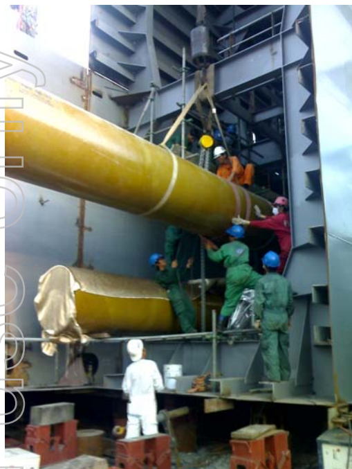
Installation of GRE pipe in the dock
