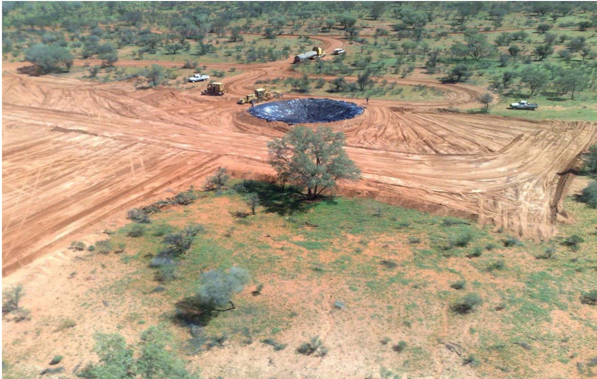
Ooraminna 2 Site Works
