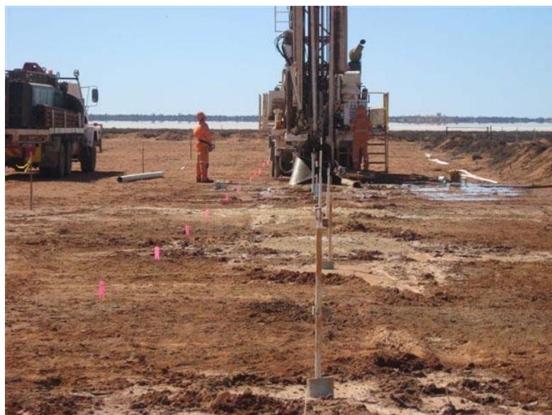
**Figure 2: Drill rig drilling water barrier lines**
