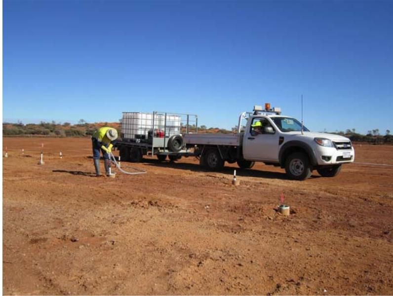
**Figure 3: Applying the geopolymers to the drill holes**
