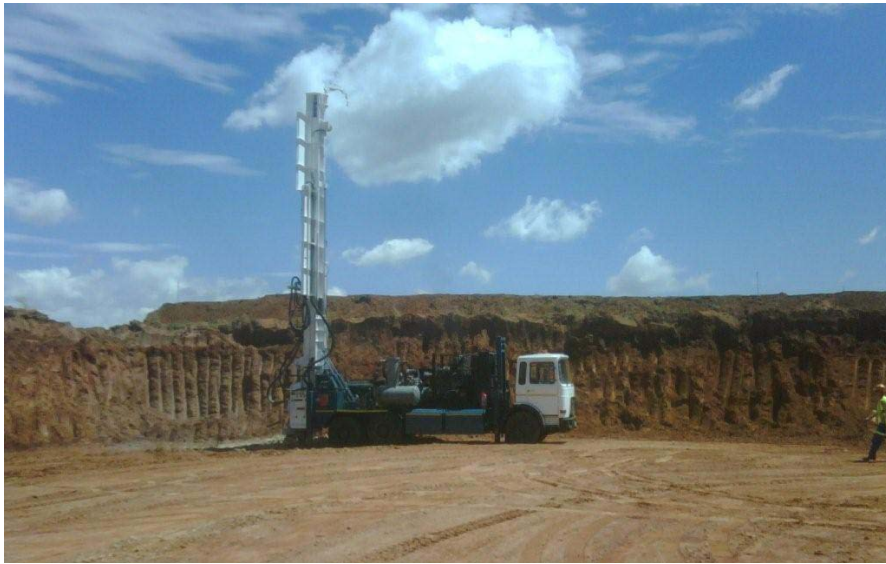
Pre-split drilling activities underway at Vlakvarkfontein
