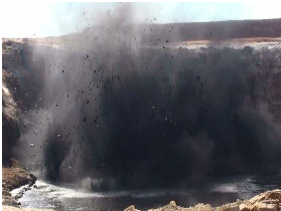
The first production blast at Vlakvarkfontein
