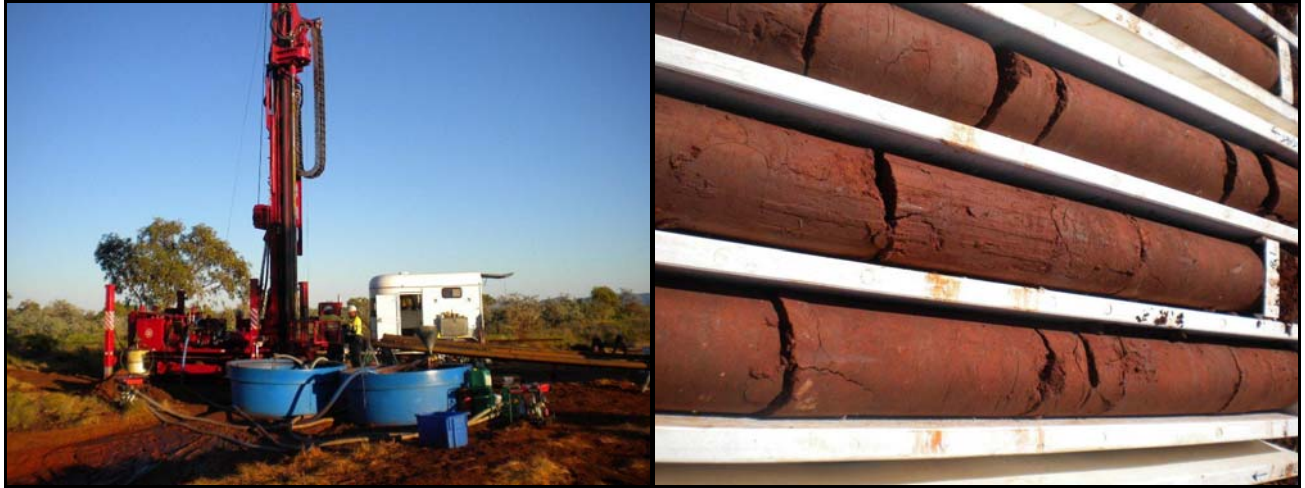
Diamond Drilling at Winmar, May 2011.
