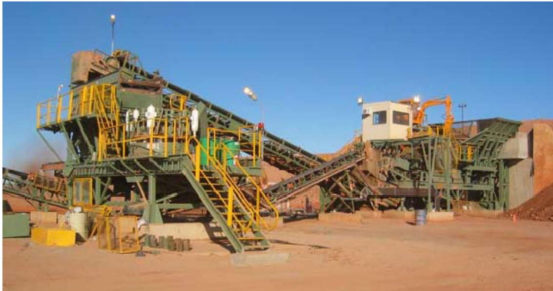
2 Stage Crushing Plant
