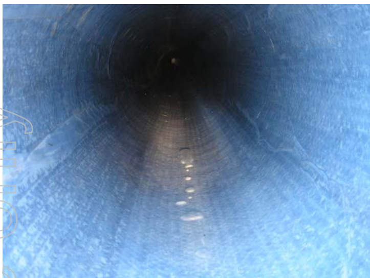
A snapshot of the finished liner
