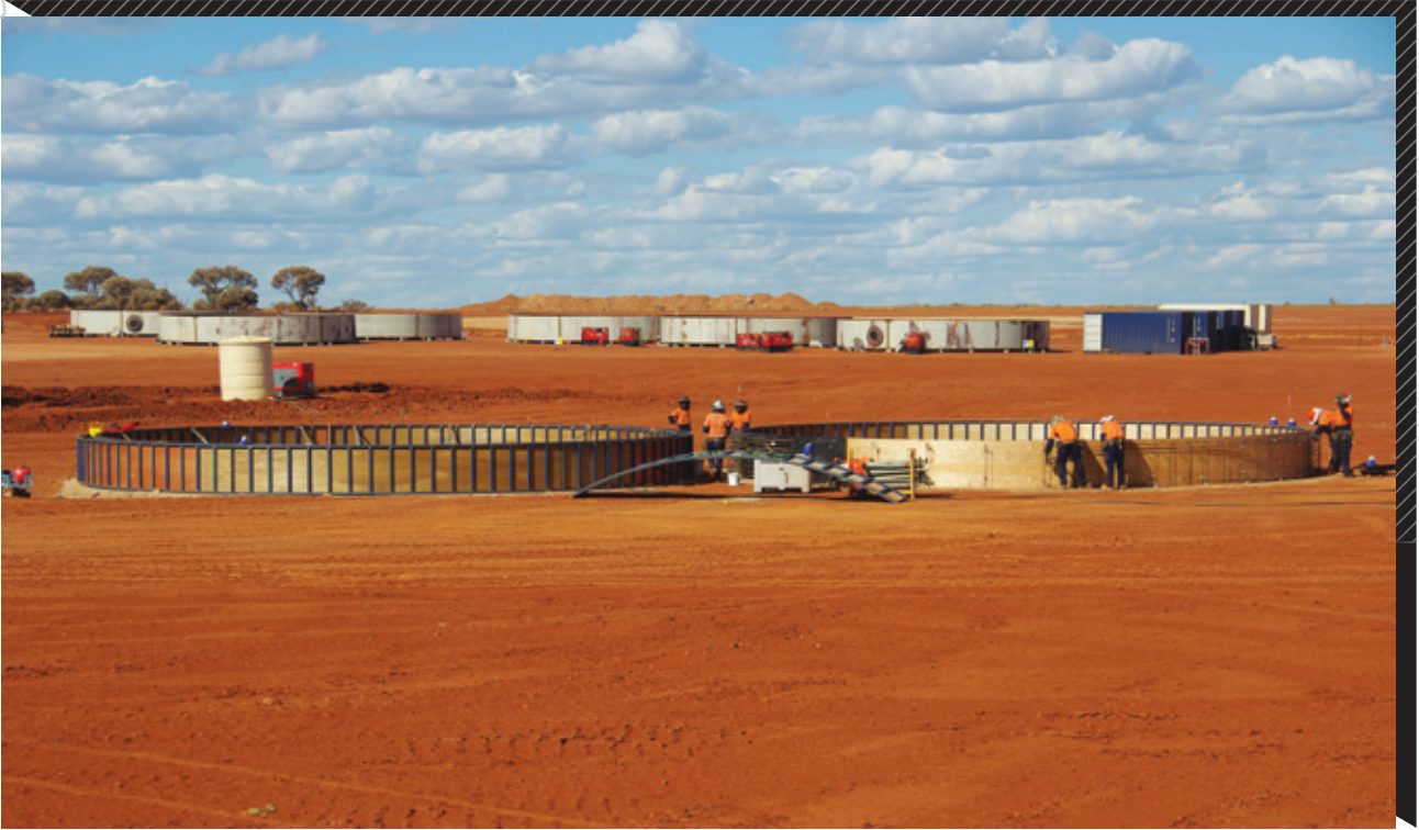
CIL tank fabrication has commenced at Garden Well Gold Project
