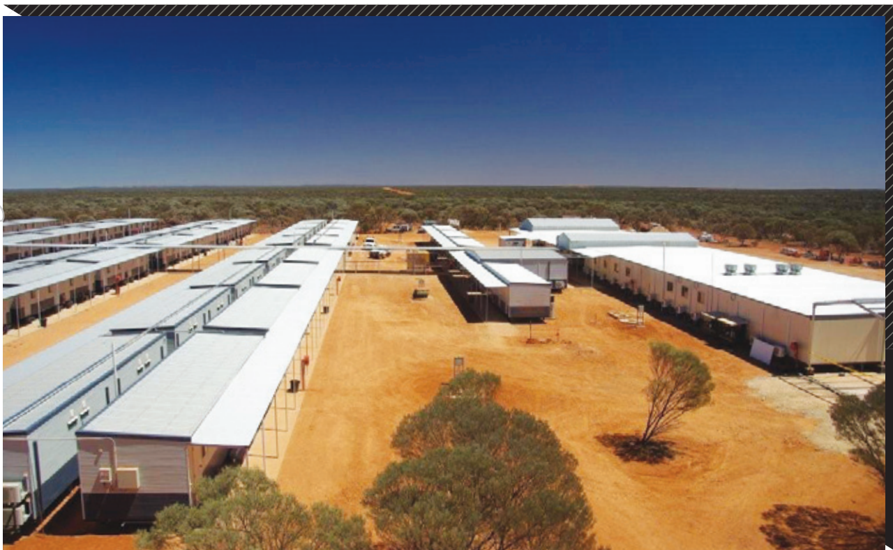
Construction of 250 man camp is nearing completion
