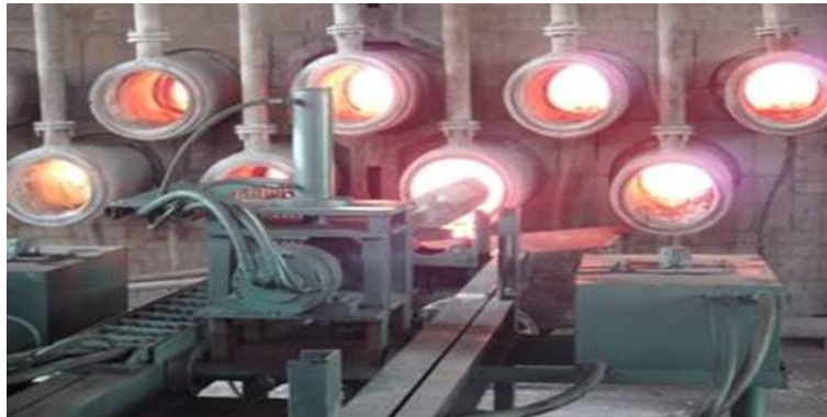
Existing furnace in production
