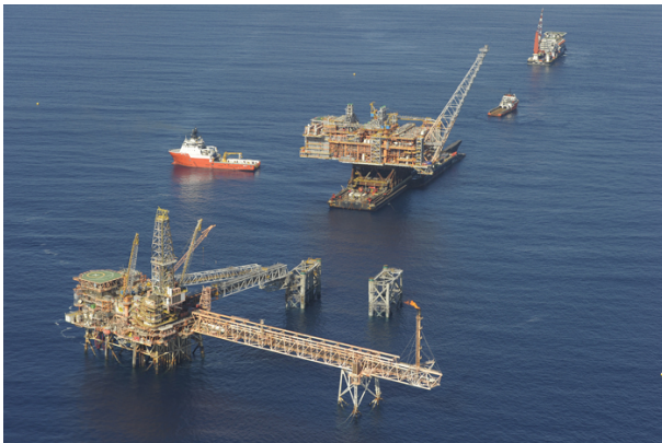
The North Rankin B topsides on Heerema's H851 barge are carried and set-down into position.
