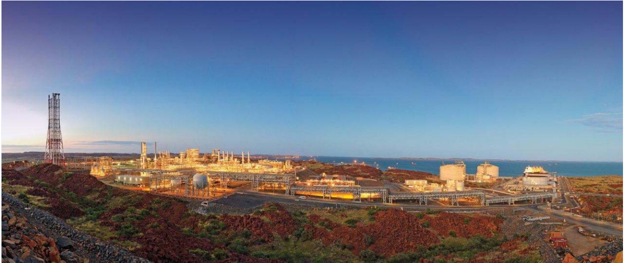
The Pluto LNG plant and associated infrastructure.
