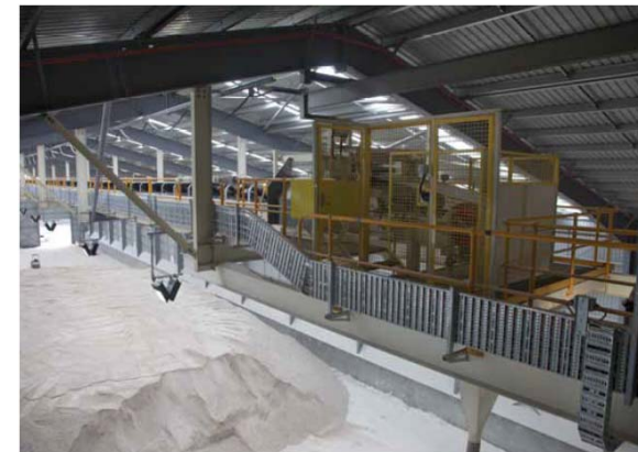
The new 40,000 tonnes gypsum store
