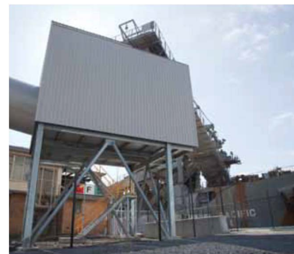
The new gypsum receiving system hopper at Wharf 26
