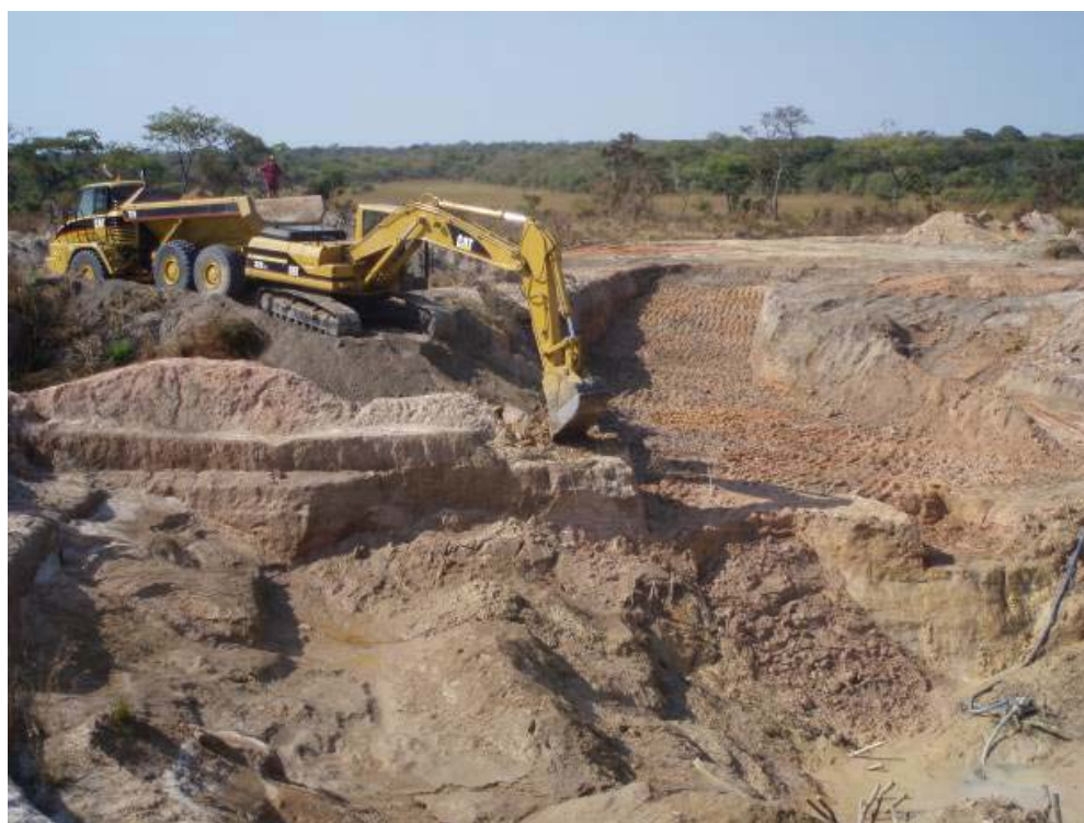
Figure 6 – Removing Overburden from Bulk Sample Pit BLK_08
