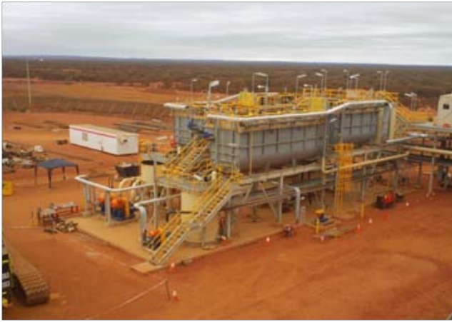
Flotation cell installation
