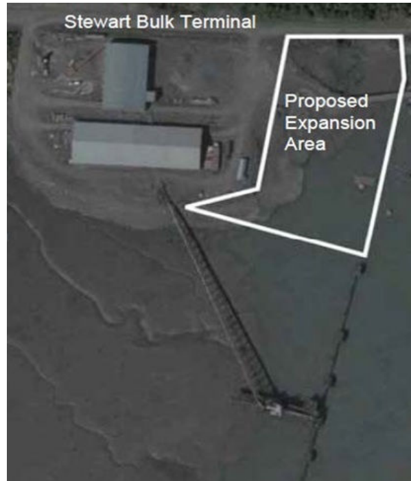
Stewart Bulk Terminal proposed expansion site
