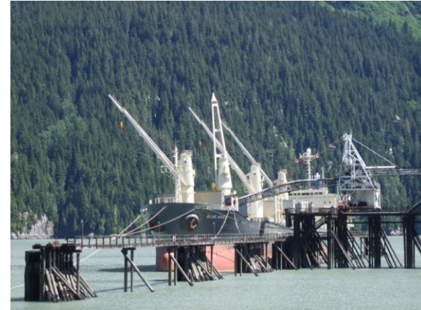
Stewart Bulk Terminal existing loading berth
