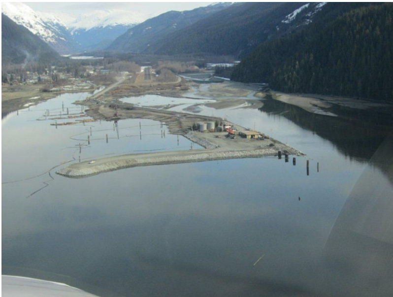
Stewart World Port dock under construction
