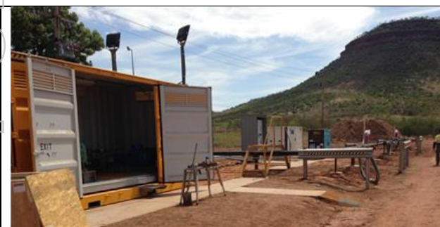
Wyndham Truck Unloading Bay
