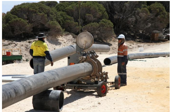
Installation of pipeline conduit onshore at Garden Island, Western Australia
