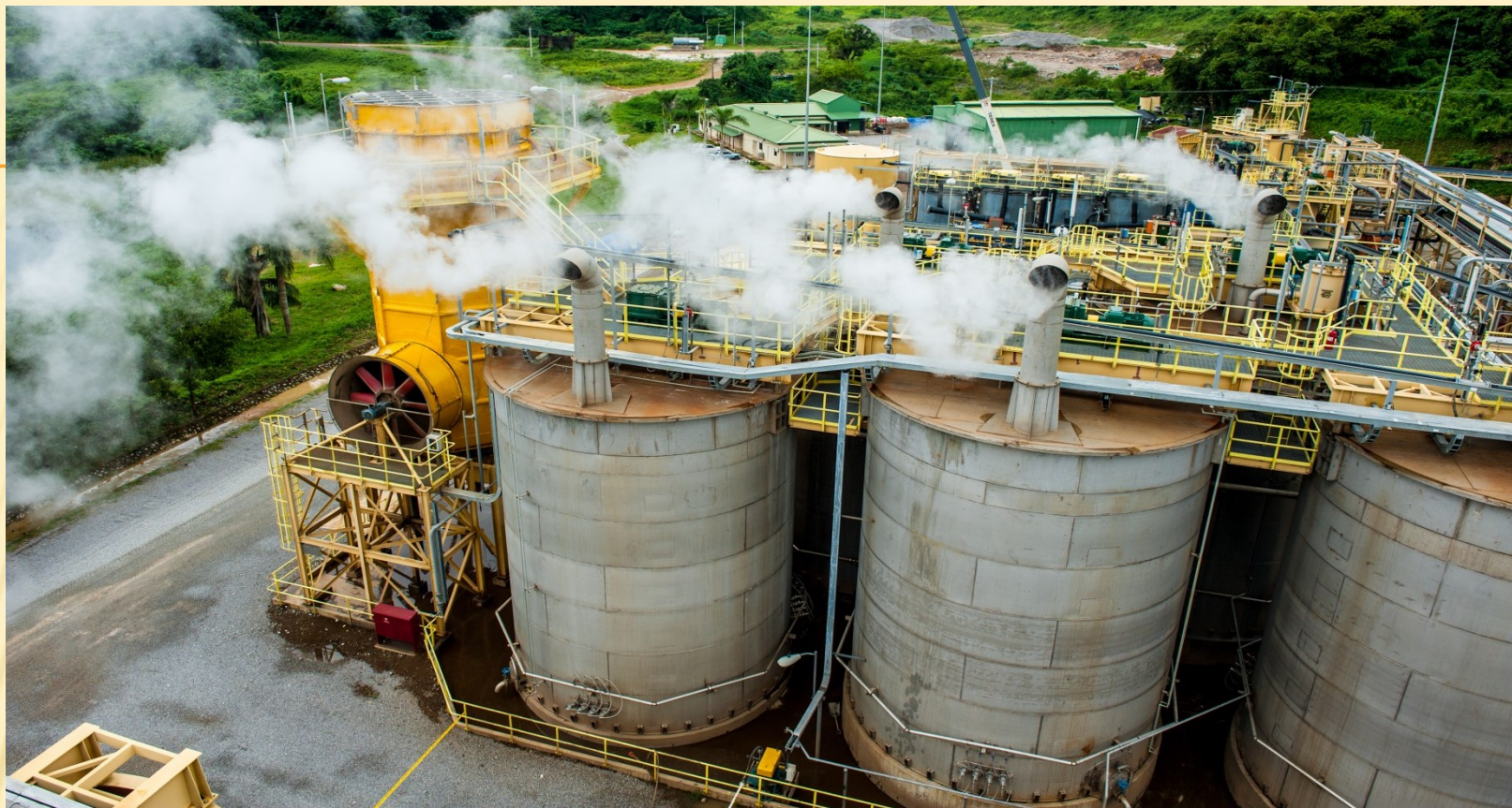
Las Lagunas Albion/CIL Process Plant, Dominican Republic
