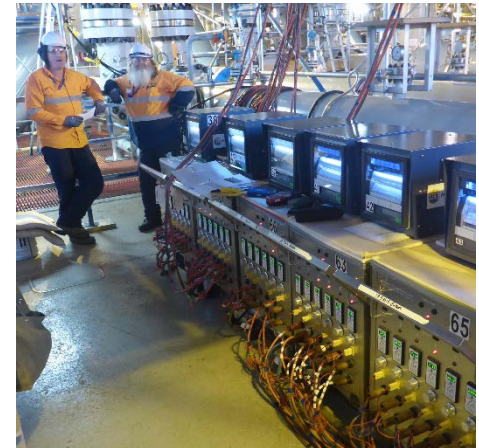
RCR Heat Treatment works on Off-shore platform for Wheatstone
