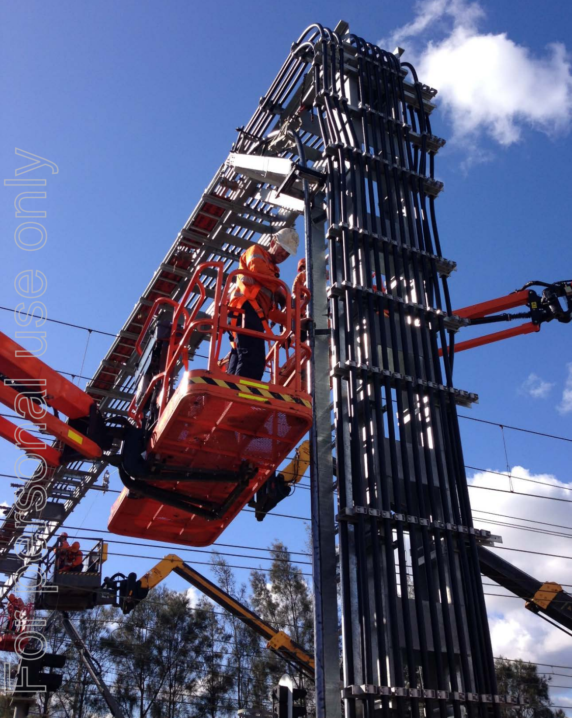
Novo Rail Alliance - Pulling HV cabling into substation, NSW
