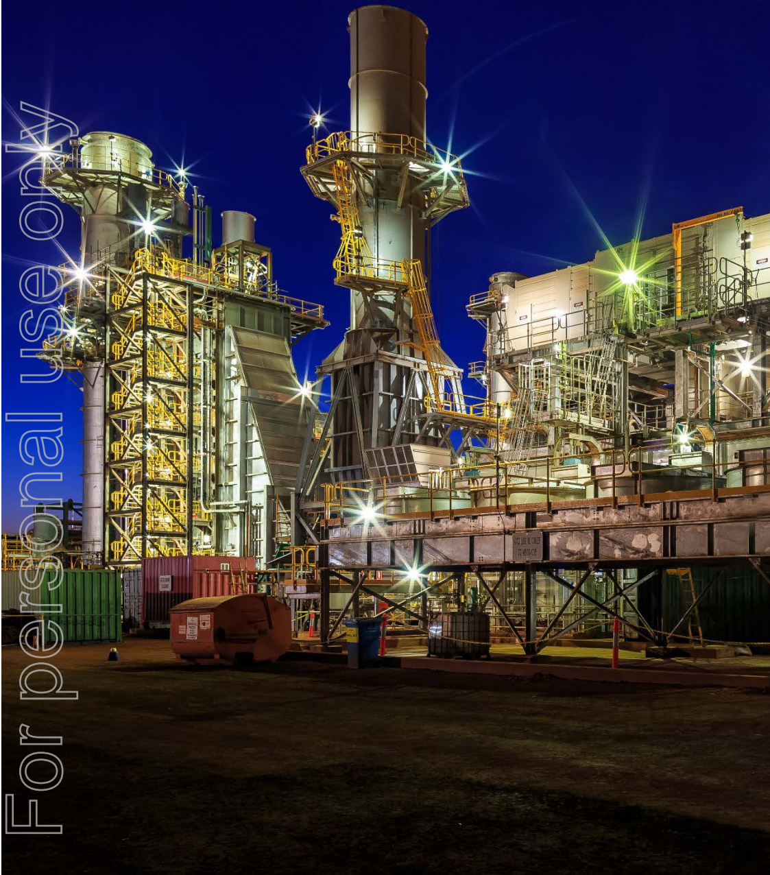
RCR designed and supplied Heat Recovery Steam Generators - Yarnima Power Station, WA
