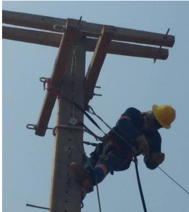
34.5Kv power cables being installed on the transmission poles
