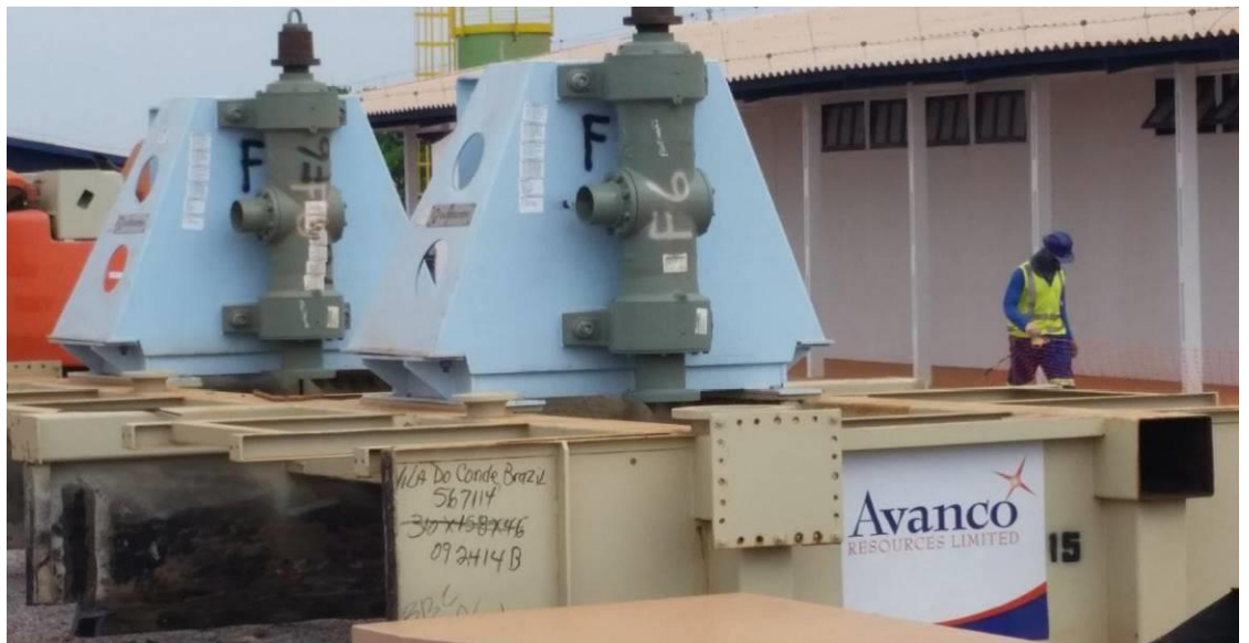
Rougher-Scavenger OK 38's Flotation Cells ready for lifting into position once the steel structures are ready
