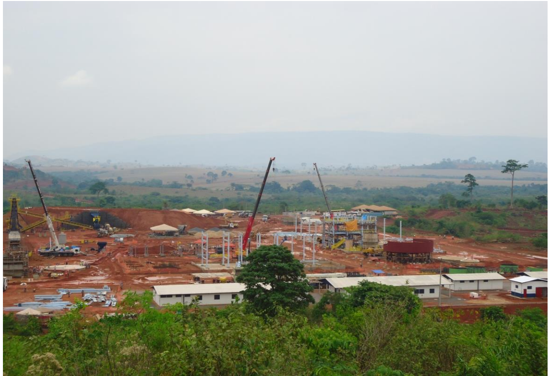
View of construction activities around the beneficiation plant
