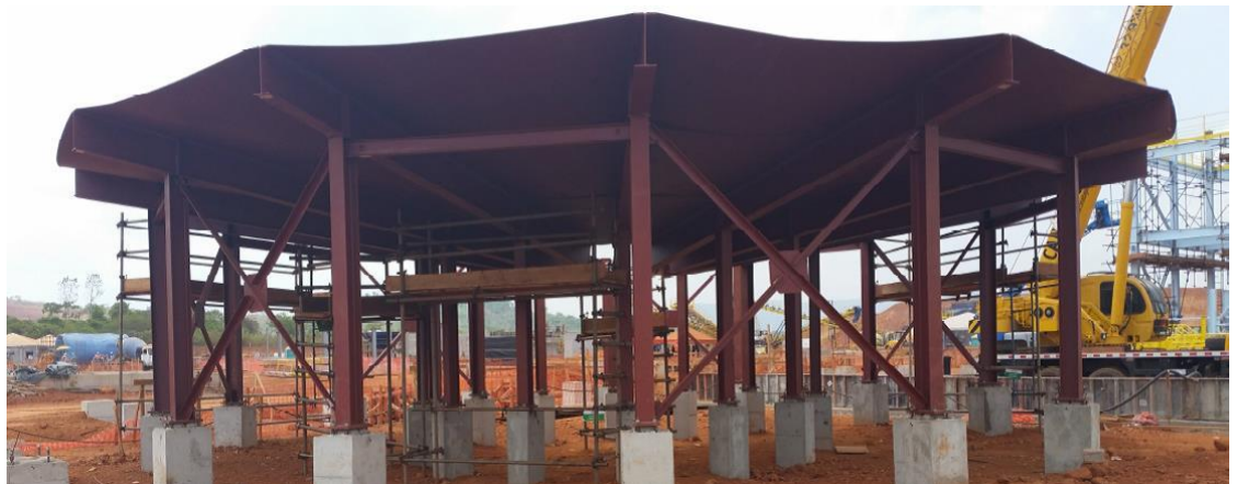
Concentrate Thickener Fabrication in Progress
