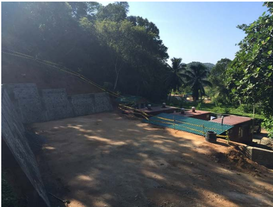
Figure 4: Shaft J Pad walls and pad site completed
