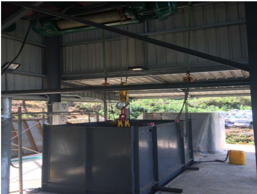
Figure 2: Box liners being prepared for lowering from hoist at Pandeniya
