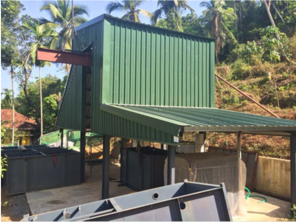
Figure 1: Pandeniya headframe and shaft box liners
