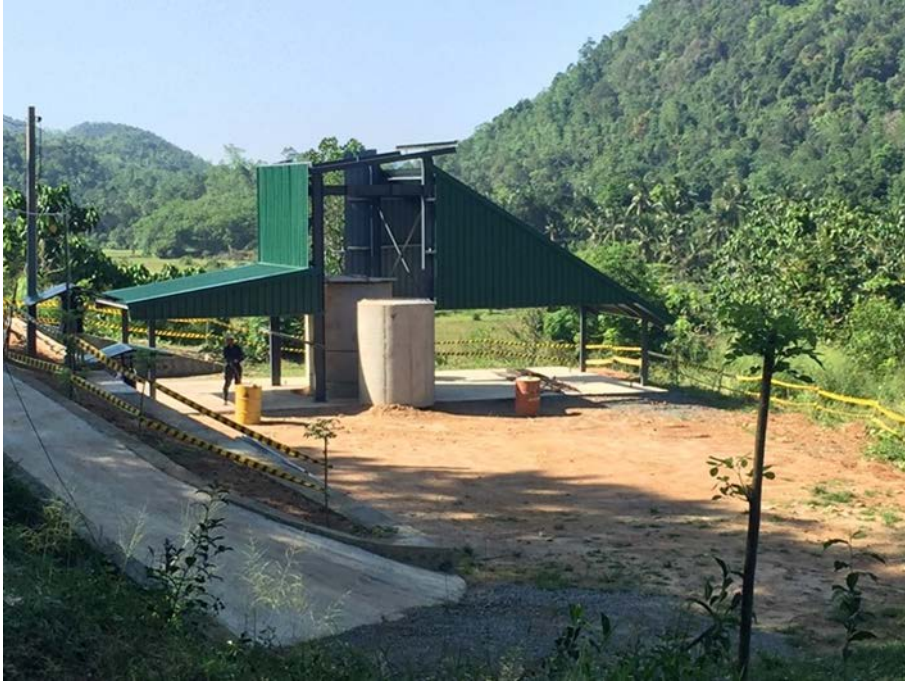
Figure 3: Shaft H Completed headframe
