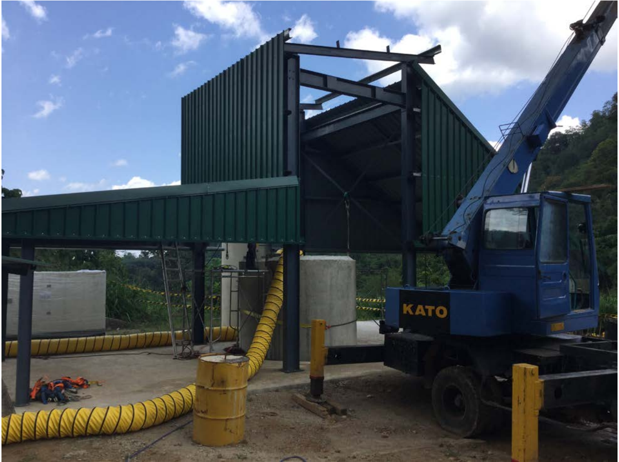
Figure 4: Shaft H Development Work
