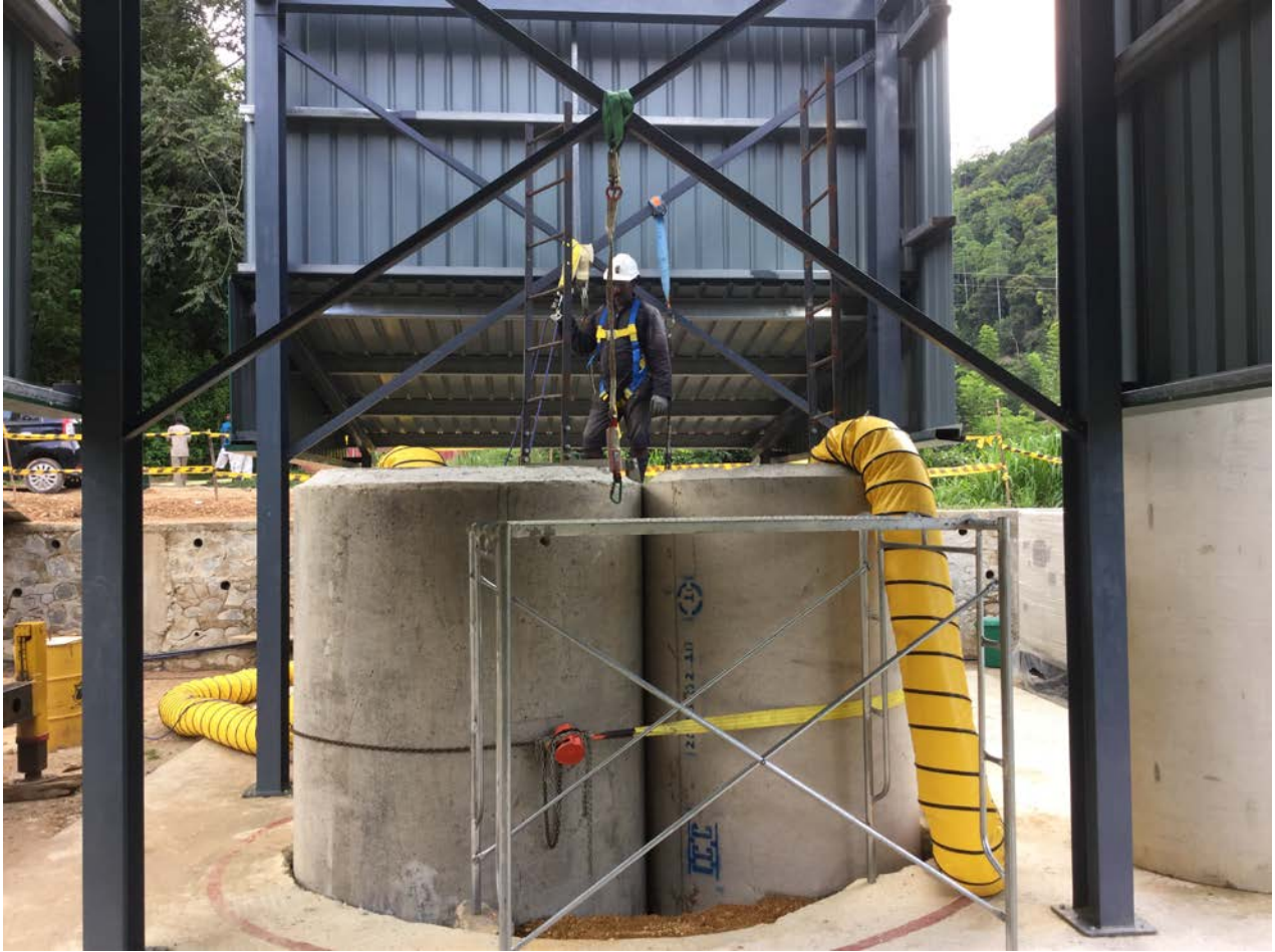
Figure 3: Sinking Liners in Shaft H
