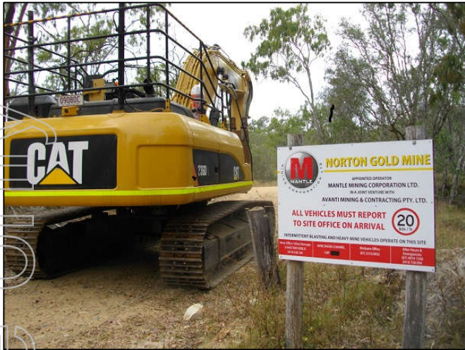
Picture 1: Mobilising to site.
