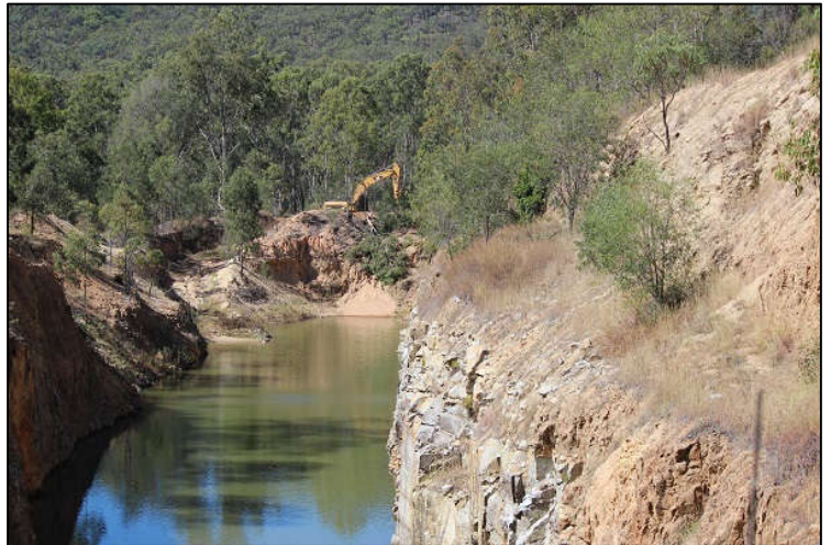
Picture 2: Excavating Never Never shear.
