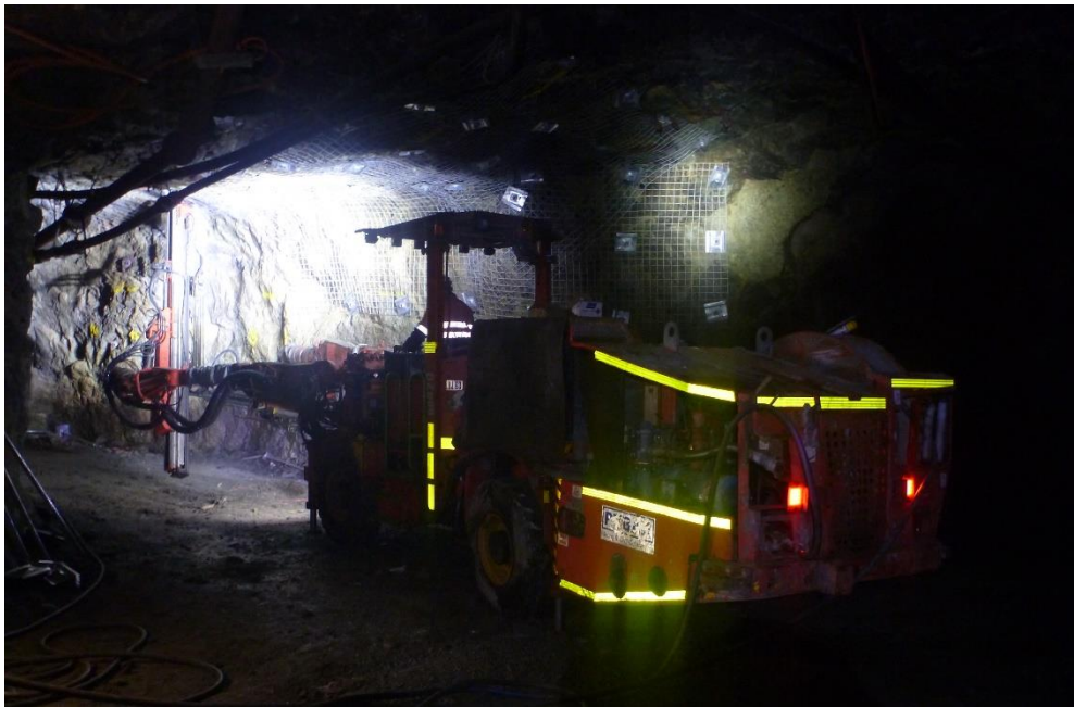
Photo 3: Pybar jumbo at work in Golden Age Pump Station
