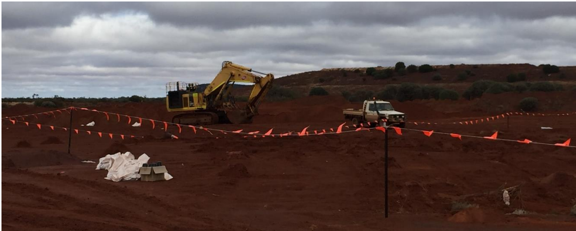
Photo 2: MACA digger at Matilda M10 pit.
